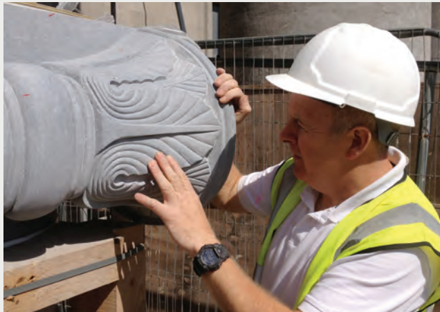
Inspecting the handcraved Limestone capital detail
