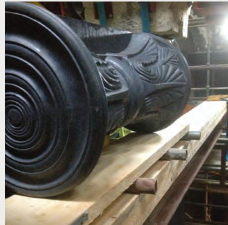
Moving the capital into place above the columns
