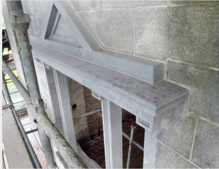
Restored window detail in solid Irish Limestone
