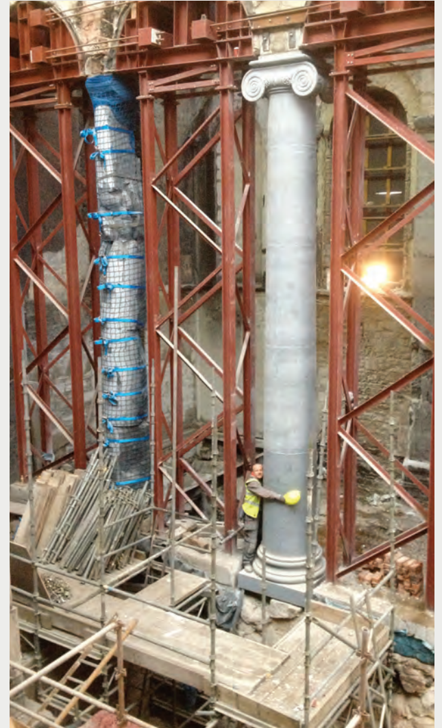
New Limestone column next to damaged column
